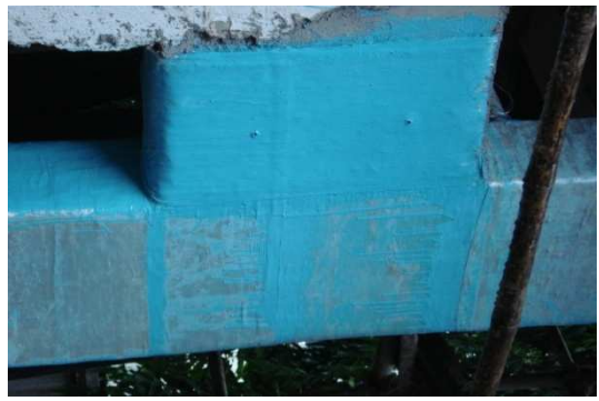
Fig 21 Strengthening of Columns and Joints using FRP Wrapping.
