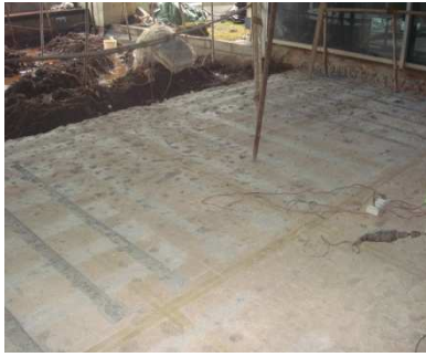
Fig 18 Strengthening of slab from above using Carbon Fibre Composite laminate with anchor plates at the end
