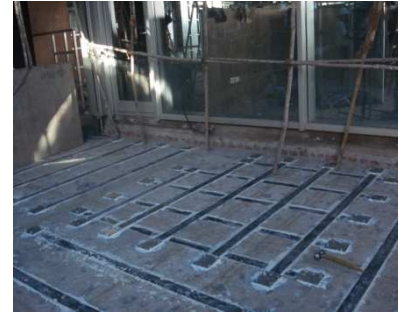
Fig 18 Strengthening of slab from above using Carbon Fibre Composite laminate with anchor plates at the end
