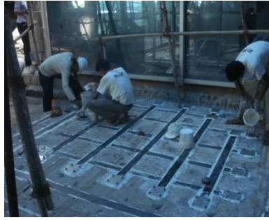
Fig 18 Strengthening of slab from above using Carbon Fibre Composite laminate with anchor plates at the end
