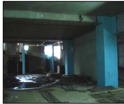
Fig 17 Fibre Wrapping of Columns to increase load capacity to fulfill the increase in design loads.
