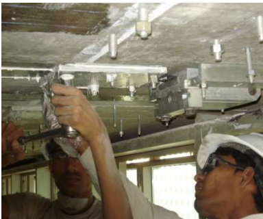
Fig 19 Strengthening of slab from below using the Pre-Stressed Carbon Fibre Laminates With anchor plates at the end
