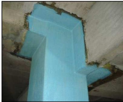
Fig 17 Fibre Wrapping of Columns to increase load capacity to fulfill the increase in design loads.
