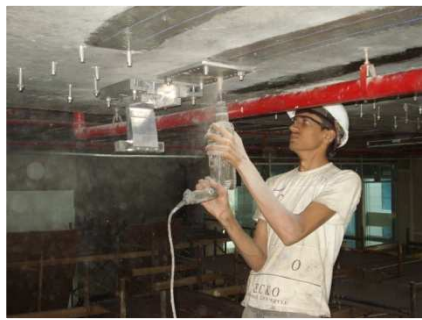
Fig 19 Strengthening of slab from below using the Pre-Stressed Carbon Fibre Laminates With anchor plates at the end
