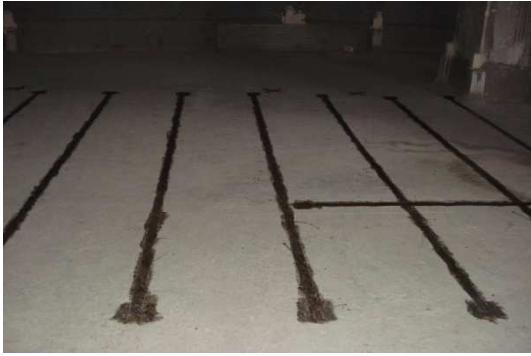
Fig 20 Strengthening with Carbon Fibre Laminate system.
