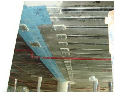
Fig 19 Strengthening of slab from below using the Pre-Stressed Carbon Fibre Laminates With anchor plates at the end
