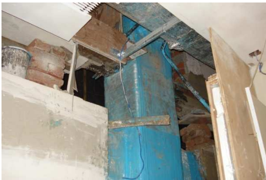
Fig 21 Strengthening of Columns and Joints using FRP Wrapping.
