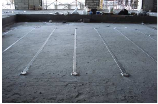
Fig 20 Strengthening with Carbon Fibre Laminate system.
